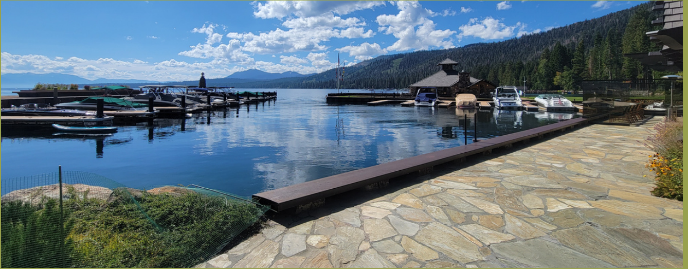
Beam repair begins at the Guard House July 2023
