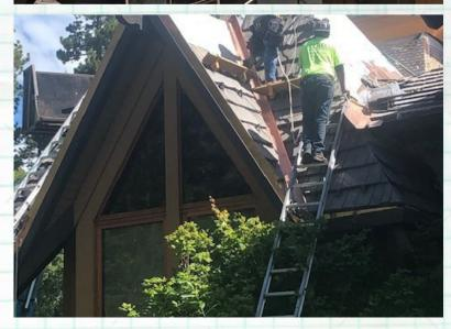
Lebel Roofing is nearing completion with roofing of the triplex 16-17-18 with only gutter and finishing yet to be done.
